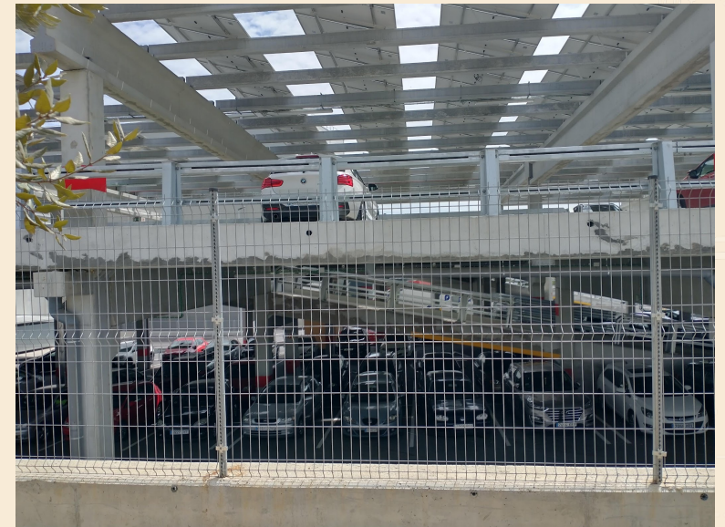
Aparcaments a Patel
